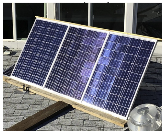
Fig. 3. Three 12 V, 100 W solar panels facing approximate solar noon (1:00 p.m. local time), receive sunlight from 9:00 a.m. to 5:00 p.m.
