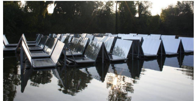
Fig. 5. V-trough solution, ( 30^\circ trough angle). FTCC system in Colignola –Pisa.
